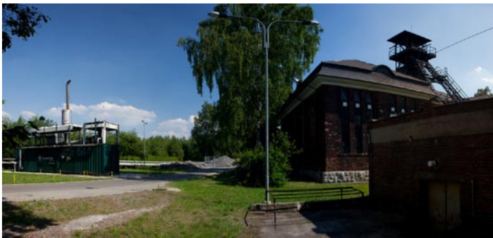
Past meets present – The Vrbice ventilation shaft and a CHP unit
